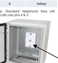
6. Secure back plate to the box using the (4) nuts ensuring phone cable is beneath the plate.
